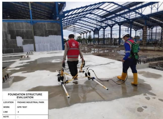
Figure 5. IDS RIS-ONE GPR equipment
