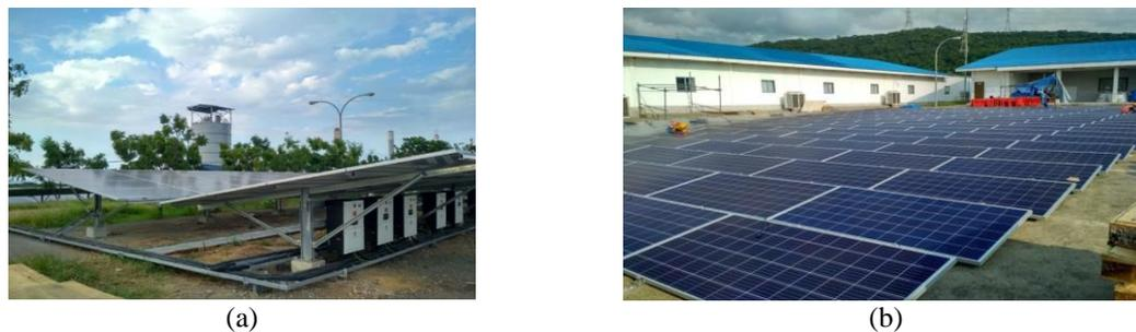
Figure 4 : (a) PV array with Ground Mounting System (GMS) instalment and (b) PV array with Ballasted Mounting System (BMS) instalment
